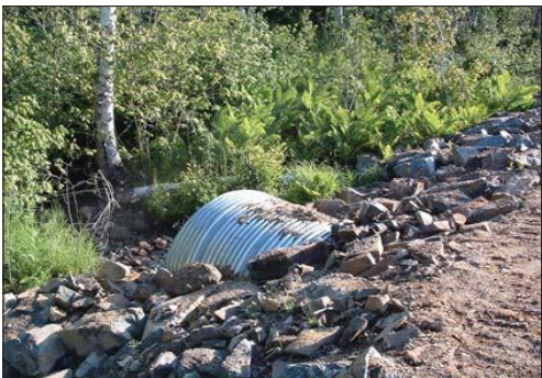
Proper use of rock for sedimentation control .
