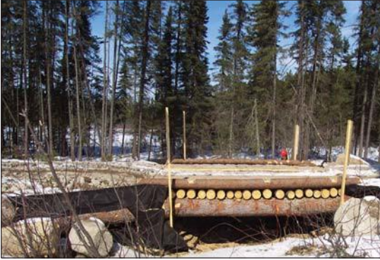
Geotextile used to prevent stream siltation.
