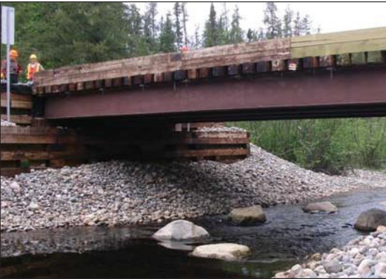
Proper sediment control on bridge structure.
