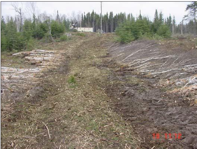
Brush mat used to cross wetland.
