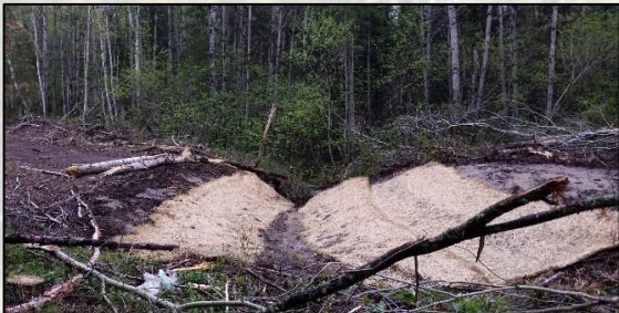
Winter crossing removal with straw mats
